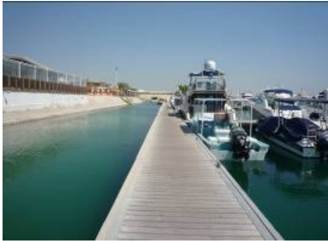
Photo 7-4: Typical Floating Berth
